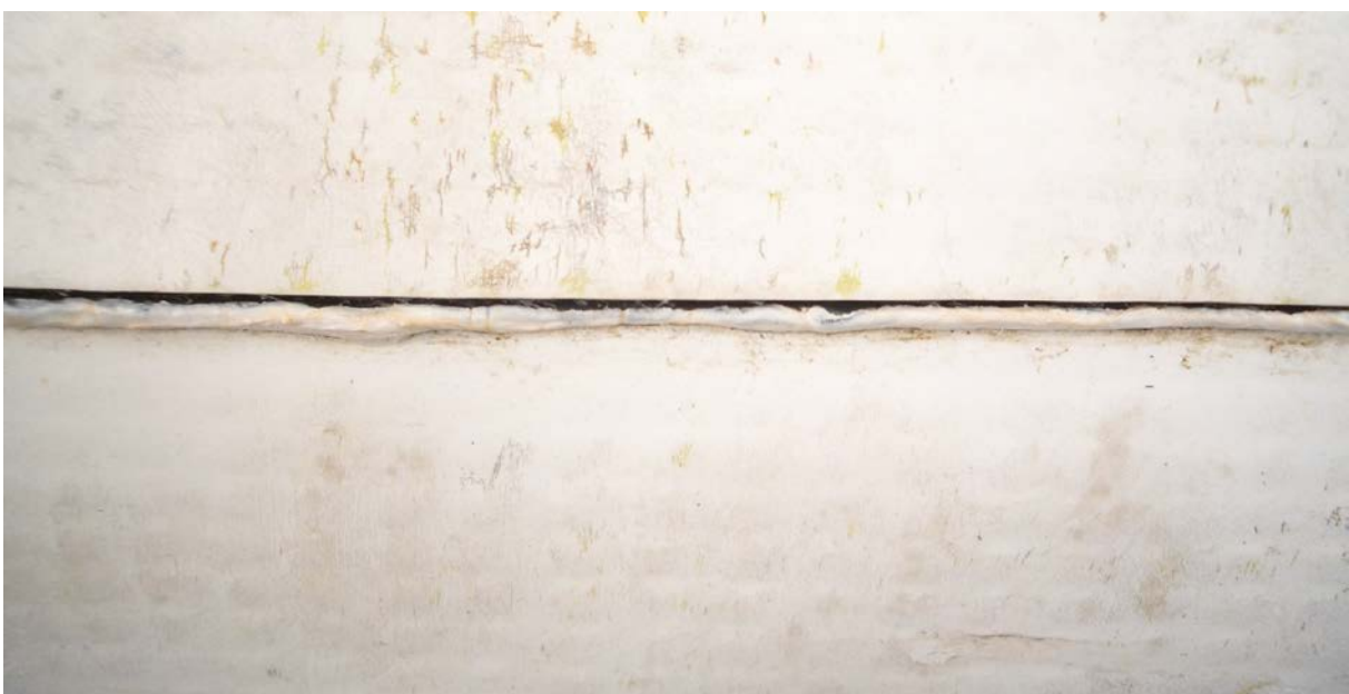
Figure 3: Sheet surface with joint (detail)
