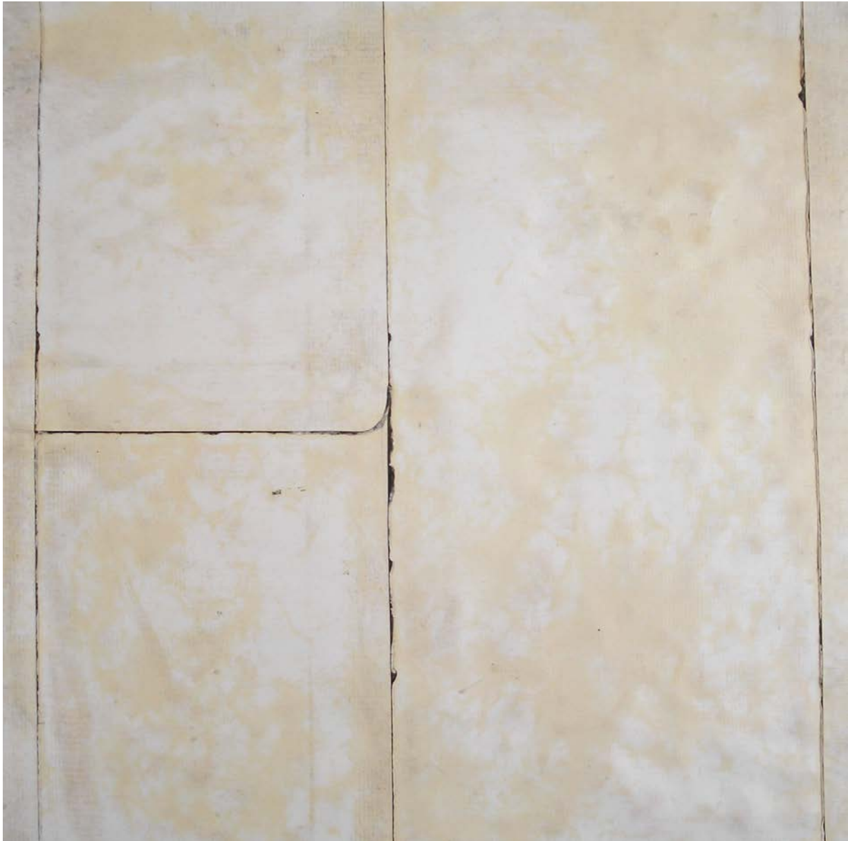
Figure 1: Sheet surface with joints
